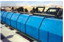
These screens operate between 75° to 81°. Three to five rakes collect the screenings one after the other and drops it on the chute about 1mtr above coping level before commencing its backward motion. These screens are fully covered.
